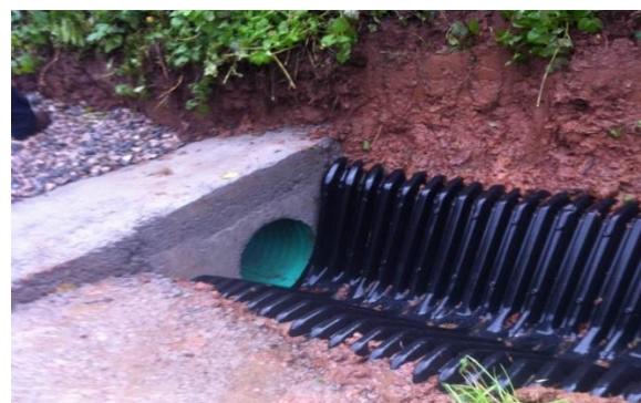
SmartDitch is sealed against the concrete face
