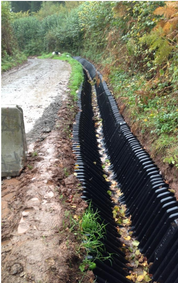
SmartDitch Installed along the side of the road
