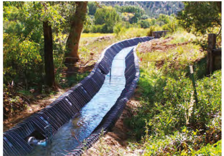
Many irrigation ditches, canals and laterals run through uneven terrain and difficult-to-access areas.
