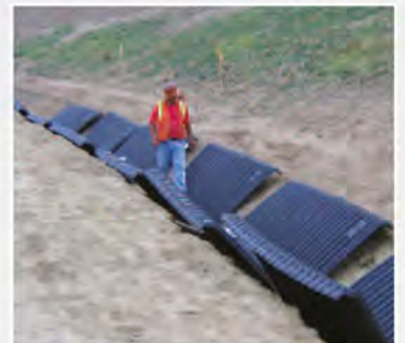
SmartDitch sections, manufactured in 8' - 10' lengths, are ready for joining.
