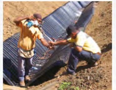
The SmartDitch anchoring system installs quickly and secures the system permanently into the ground. Earthen and concrete anchoring systems are available.
