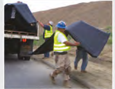
SmartDitch is light enough to be hand-carried to the damaged ditch area. No arduous ditch preparation or sandblasting is necessary prior to installation.
