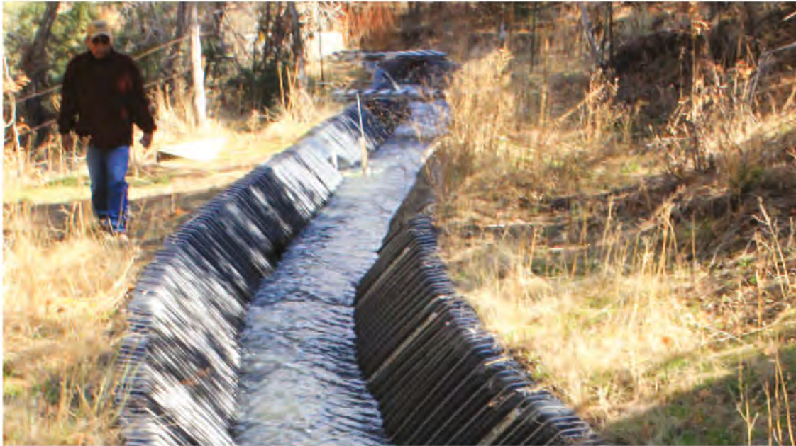
Ditch Bosses walk the ditches every day in rural farming communities. They make sure the ditches are maintained, that the farmers are getting their fair share and the water remains protected and clean.
