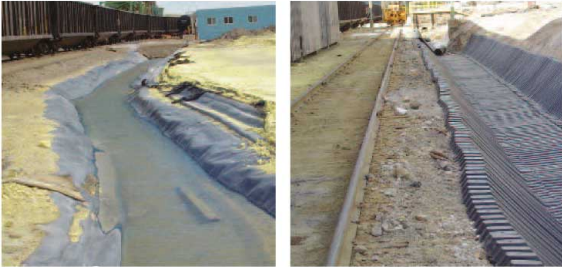
SmartDitch was the ideal channel design solution to protect the land from chemical infiltration and direct the water and chemical discharges to a containment area.
